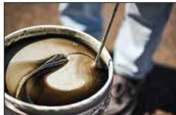
Combine Part A with Part C, then mix with Part B to a smooth consistency using a slow-speed mixer.
