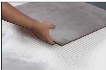
Position tiles within open time, press firmly with a slight twist and adjust using a rubber mallet.
