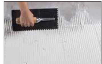
Spread adhesive with a notch trowel. Maintain a 3-12mm thickness based on tile dimensions.
