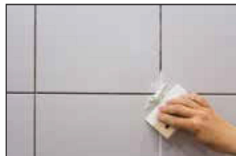
After 24 hours, remove spacers, fill gaps with Ramco Epoxy Tile Grout and wipe excess grout with a damp sponge before it dries.
